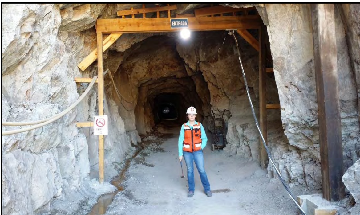
Photo 7-6: Main Portal at Babicanora, 4 m by 4 m, Built in the 1860s
