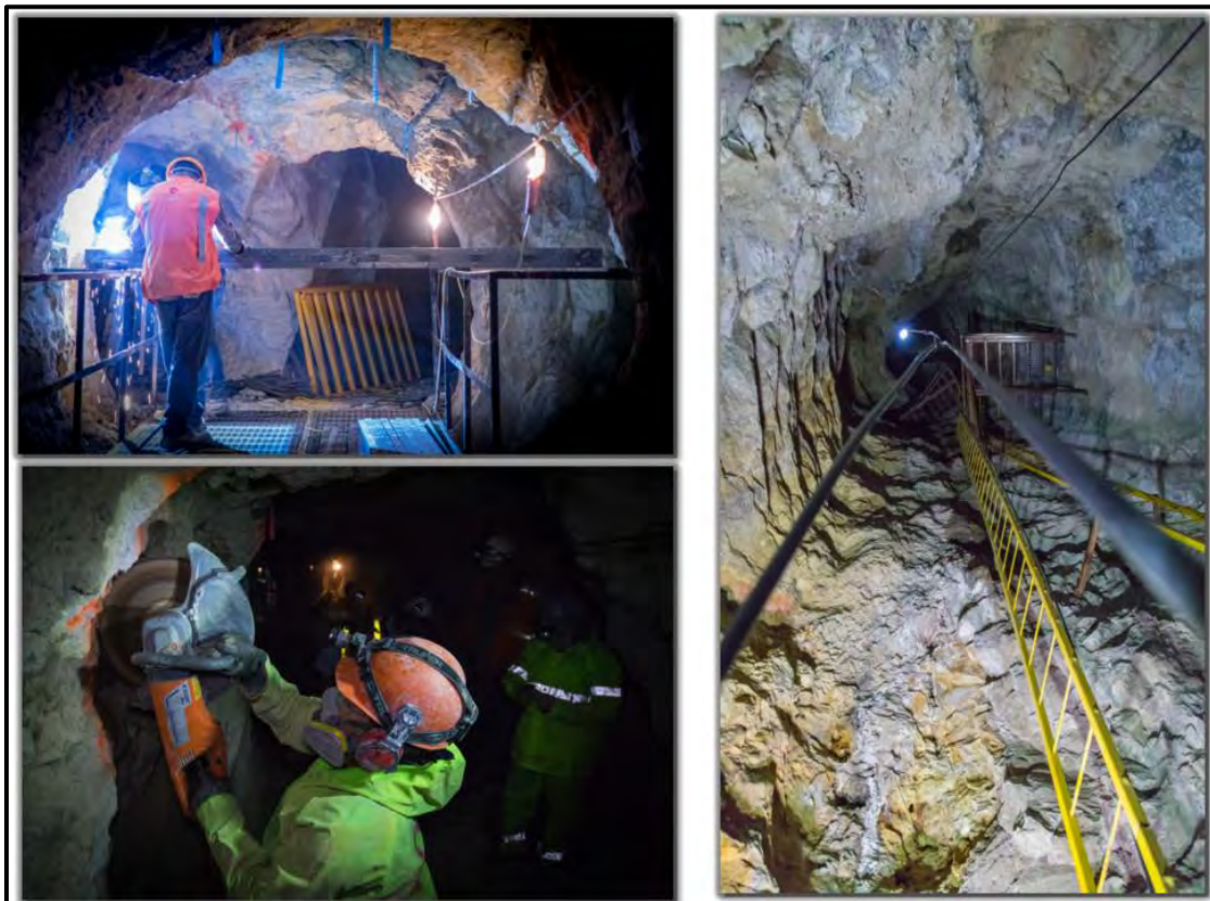
Photo 9-1: Photos of Las Chispas Underground Rehabilitation Activities
